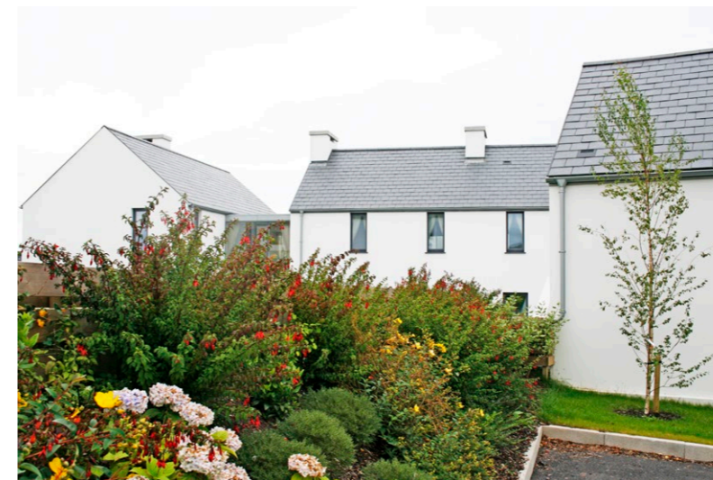
The boundary between dwellings is demarcated by a new ditch, planted with wildflowers and native shrubs. Reference: Waterfall, Co. Cork, O'Mahony Pike Architects
