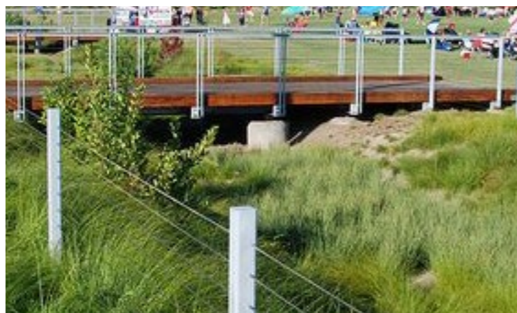
Pedestrian bridge over watercourse
