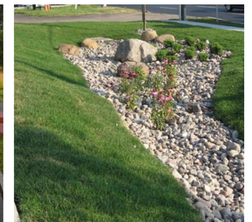
A depression which can attenuate water when required
